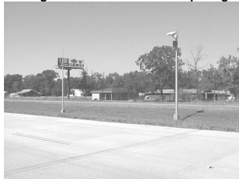
Camera Equipment for WIM - Records Picture of Truck as it Passes WIM Monitoring
